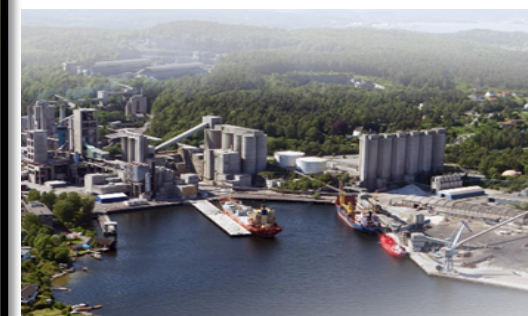
Norcem, Cement production
