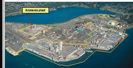
Yara, Ammonia production
